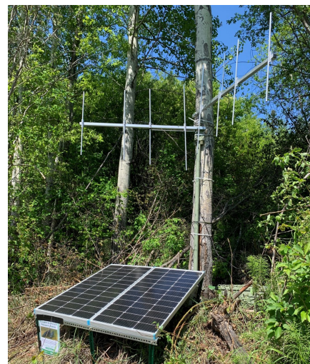
Figure 7: Radio receiver station deployed at rkm 191.
