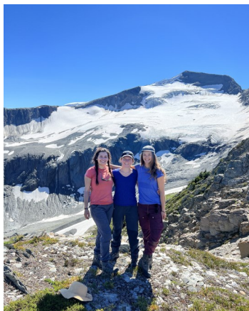
Left: The field team after dismantling the old radio repeater on the ridge above Castle Glacier
