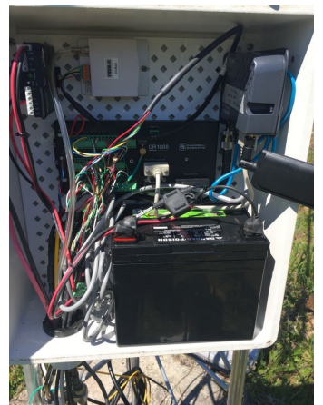
Figures 1 & 2: Weather station wiring at the Aleza Lake site. The upper left picture contains the old battery, whereas the lower right picture contains the new battery. Note the shifting of components and electrical tape on the battery terminals in the latter picture.
