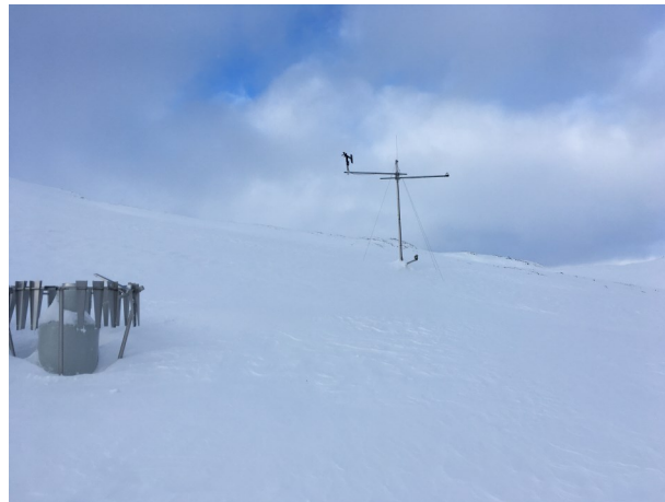
Mt Sweeney weather station covered in snow, 8 February 2021 Photo courtesy of Scott Klassen
