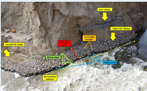
Aerial view of key "nature-like" fishway features which will support fish travelling upstream. Photo: DFO
