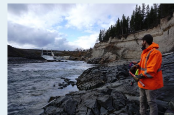
Jeremy Morris seen here pondering how to anchor the data logger downstream of the Skins Lake Spillway knowing that flows next spring will be 10 times what they were on the day of installation.
