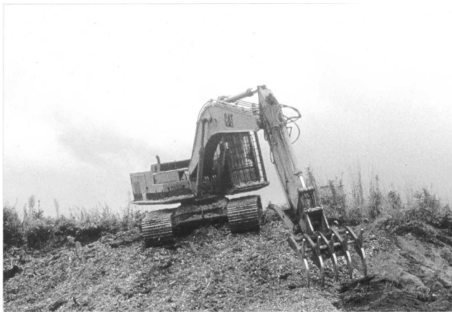
Figure 3. Site preparation rake attachment, mounted on hydraulic excavator, being used to incorporate waste wood chips.
