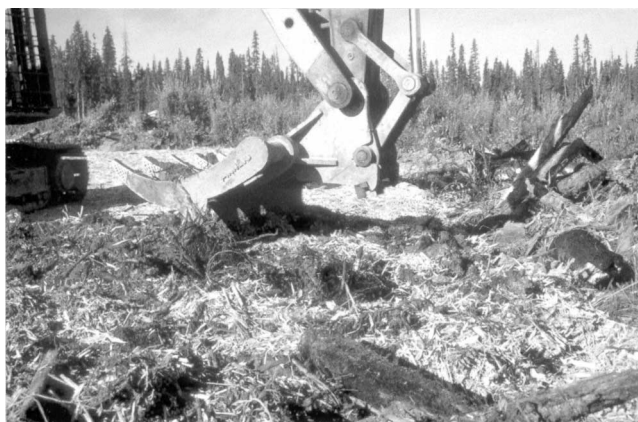
Figure 4. Close-up of incorporation of 10- to 15-cm layer of waste wood chips into upper 30–35 cm of surface soil on fine-textured landing (July 1996).
